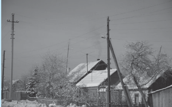
FIGURE 12.5 Power lines near houses. (Used with permission from © Diana Ninov/Alamy.)
